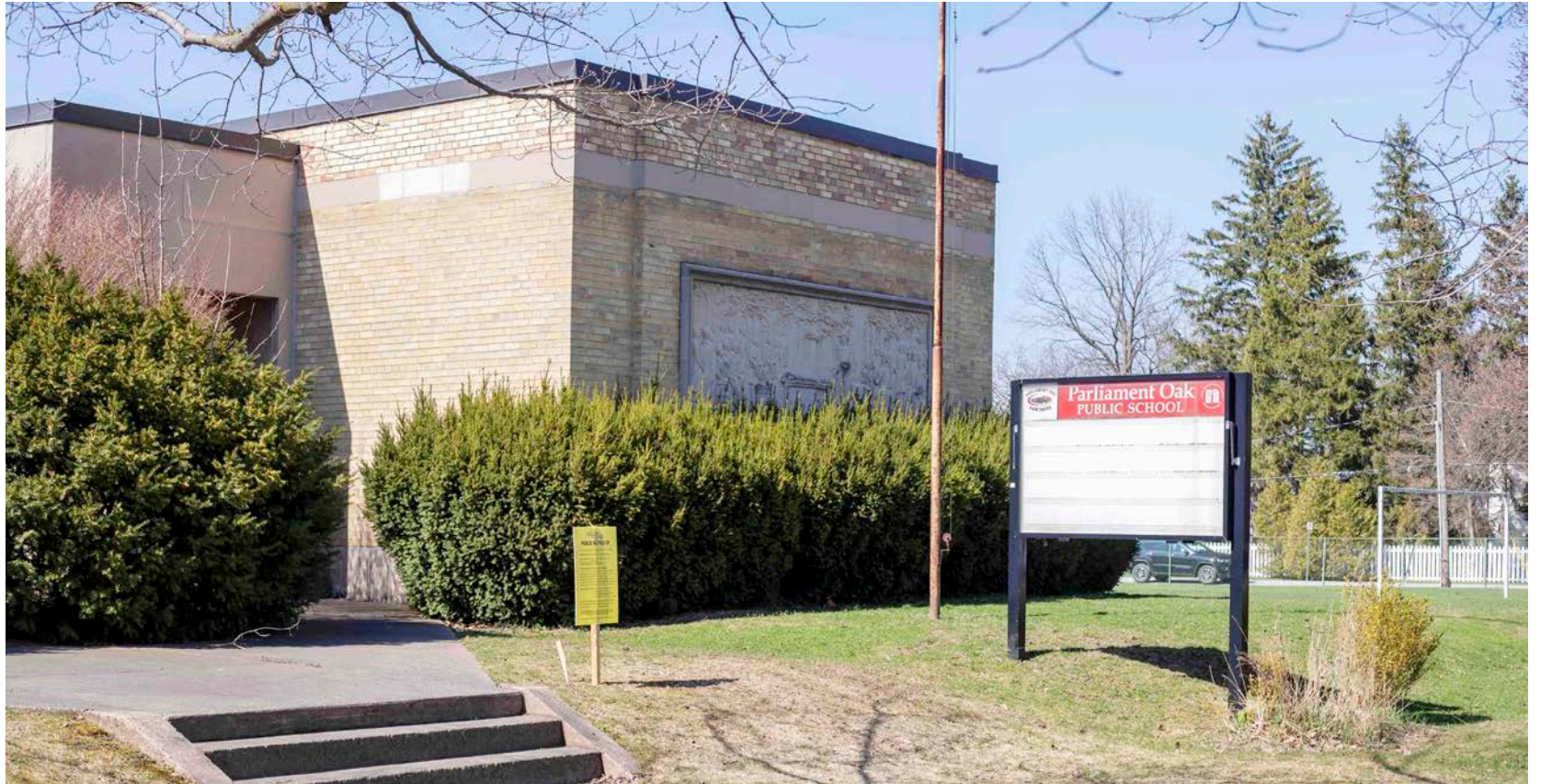
Two Sisters Resorts Corp. has plans to demolish the old Parliament Oak school with intentions to preserve some of its heritage features EVAN LOREE
